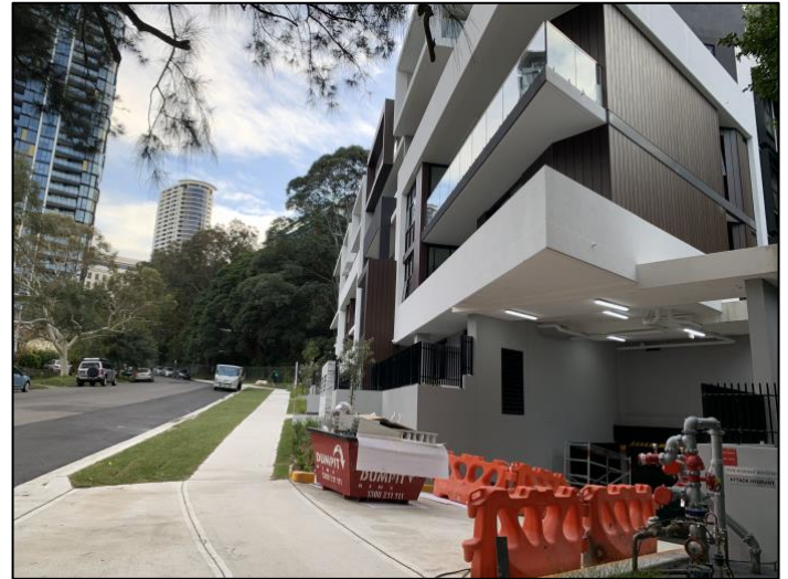
Figure 6 – Flat Building Along Duntroon Ave Looking North Source: Mecone
