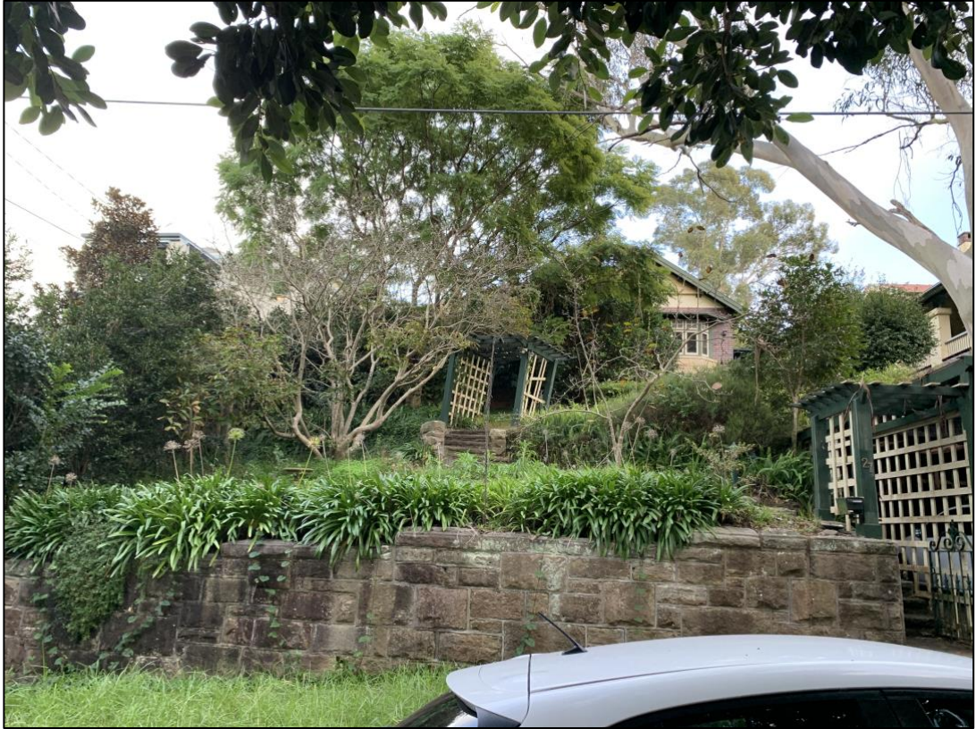
Figure 3. Dwellings Along Canberra Avenue Viewed Looking North Source: Mecone
